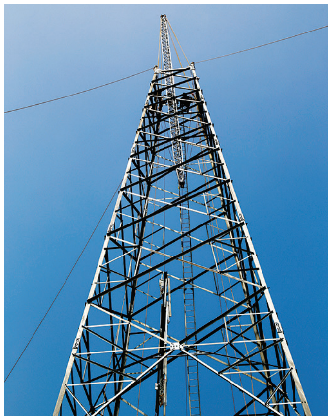
4. Using the Ginpole as a centrally placed floating Ginpole.
