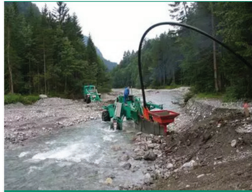
Laying system on rocky ground
