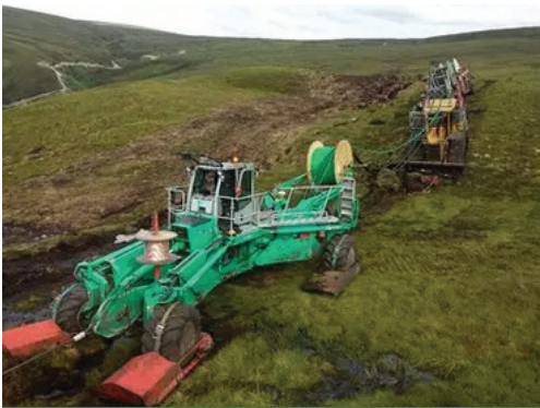
Laying system in mud and bog areas
