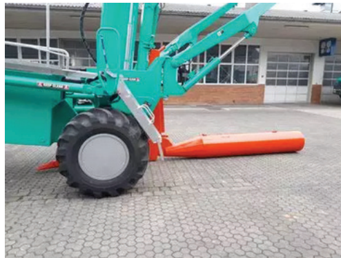
Laying steel pipes using the torpedo plow method
