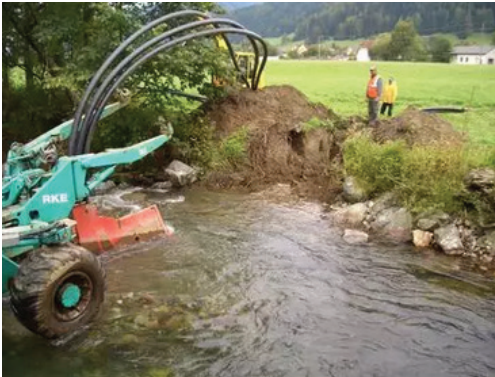
Laying pipes through watercourses
