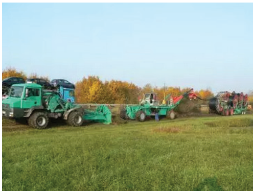
Laying of power cable
