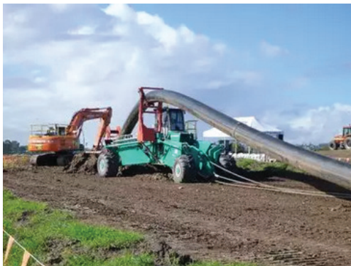
Laying of gas- and waterpipes
